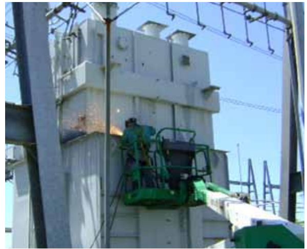
Removing the Top of the Transformer
