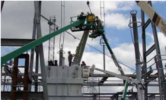
Preparing to Remove the Bushings
