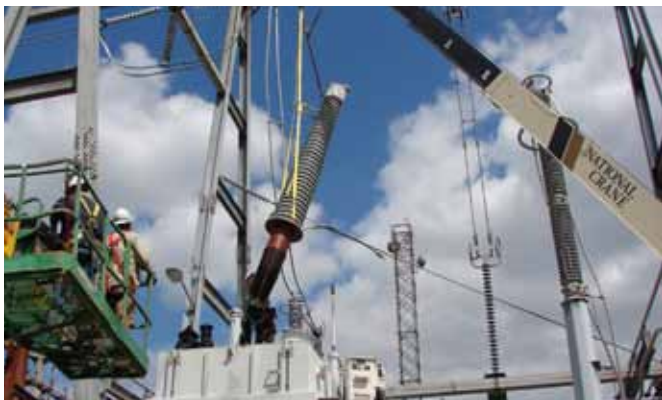
Transformer Bushings are Removed
